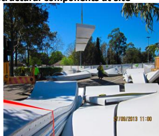
Structural components at site
