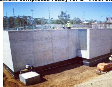
Basement completed ready for 1 st Floor slab
